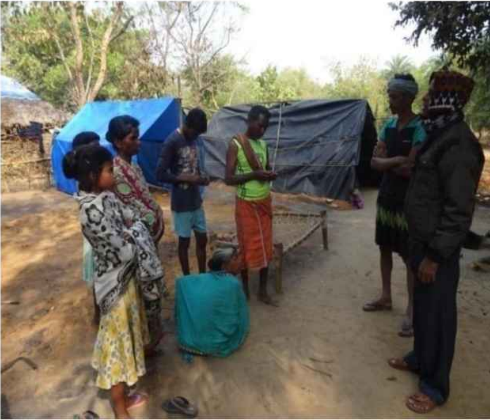
HOUSE CONSTRUCTION AT JHATIODA
